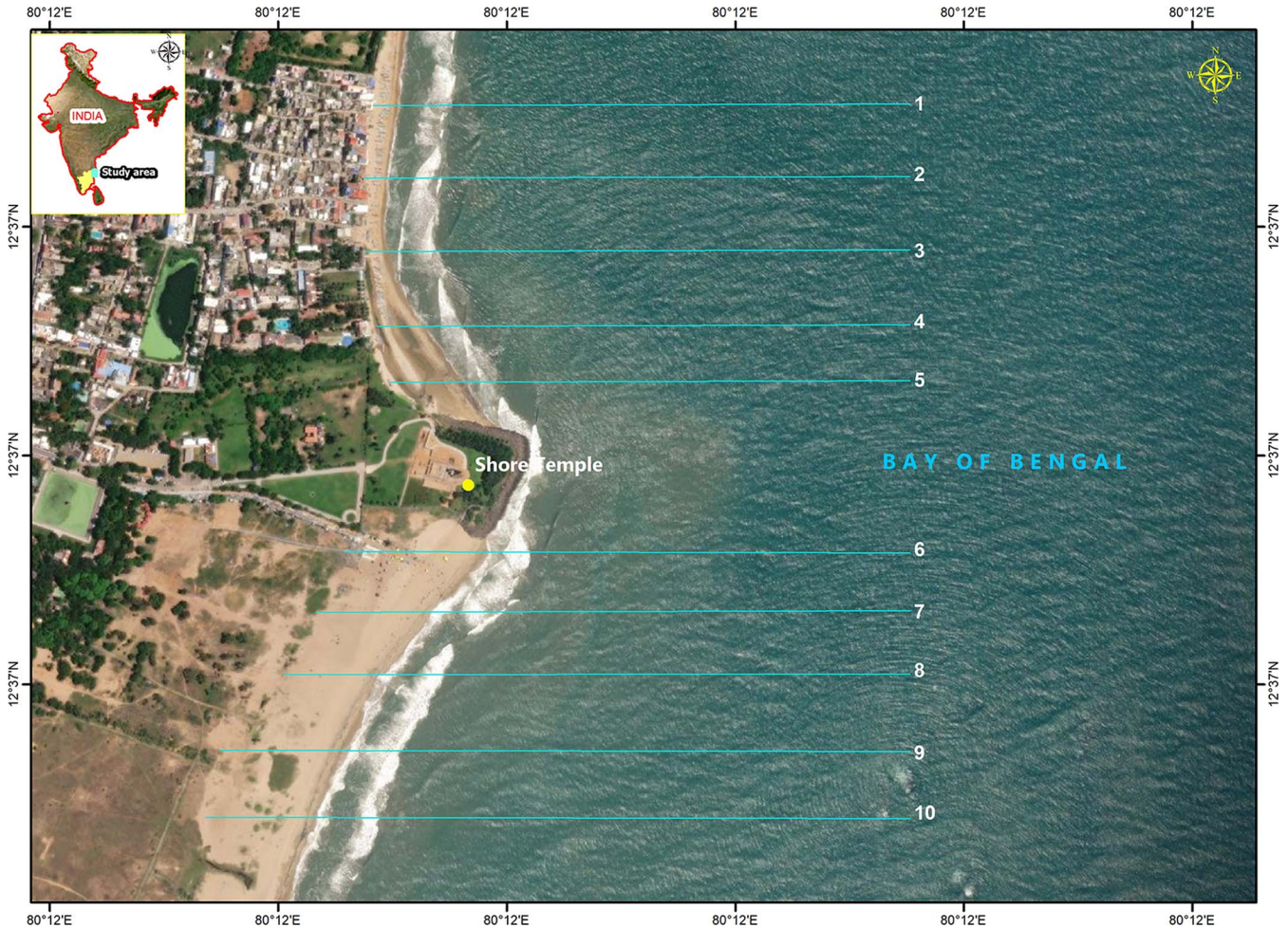
Figure 2. The present study considers transects numbered from 1–10. A shore-protection structure at the center of the study area divides it into north and south sections. Transects 1–5 cover the northern section, whereas transects 6–10 cover the southern section of the study area.
