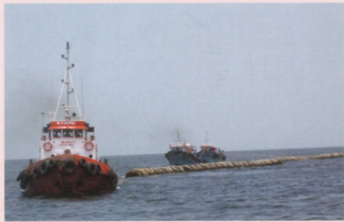
Laying of Pipelines
